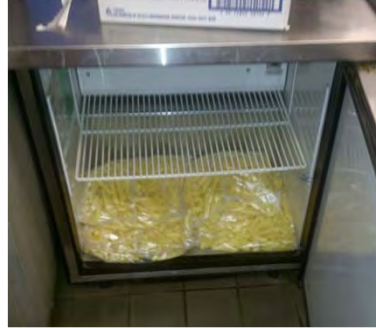
Reach-ins have temperature stratification & fluctuations
