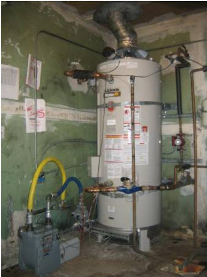
*Figure 1. Water Heater in FSR #1 – Dublin, CA*
