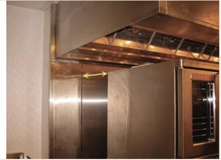
are not necessary.” They are! In our experience, the C&C performance along the end of the hood is always improved by adding a panel or skirt. Alternatively stated, a high-performance hood with end panels becomes an even higher performing hood than it is in its naked configuration.
