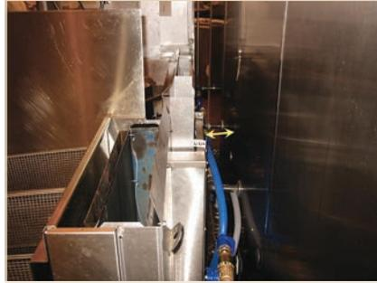
PHOTO 3 (LEFT) AND PHOTO 4 (RIGHT) Real-world illustrations of excessive gap behind cooking equipment and wall.
