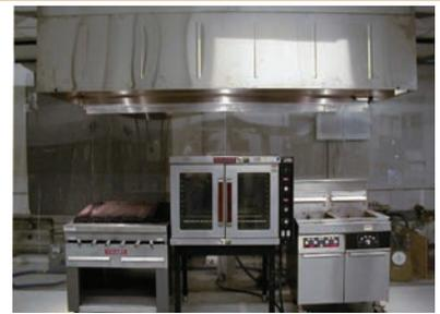
PHOTO 7 (LEFT) AND PHOTO 8 (RIGHT) Illustration of heavy-duty appliance position under a wall-canopy hood.
